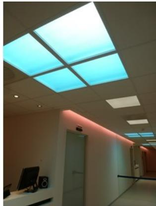
Figure 1 Philips BlueSky mimicking a blue sky view and sunny daylight for environments with limited real daylight
