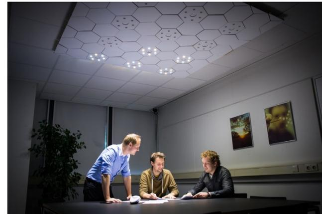
**Figure 1** A meeting room intelligent lighting installation featuring Hyvve, a hexagonal light tile with computation and wireless communication capabilities (design by Remco Magiels, TU/e Industrial Design).
